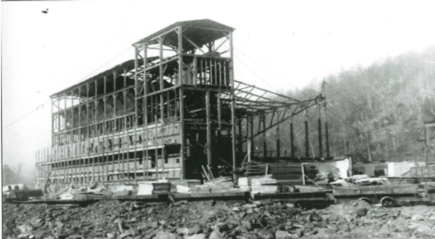
Vinton #6 Washery under construction
