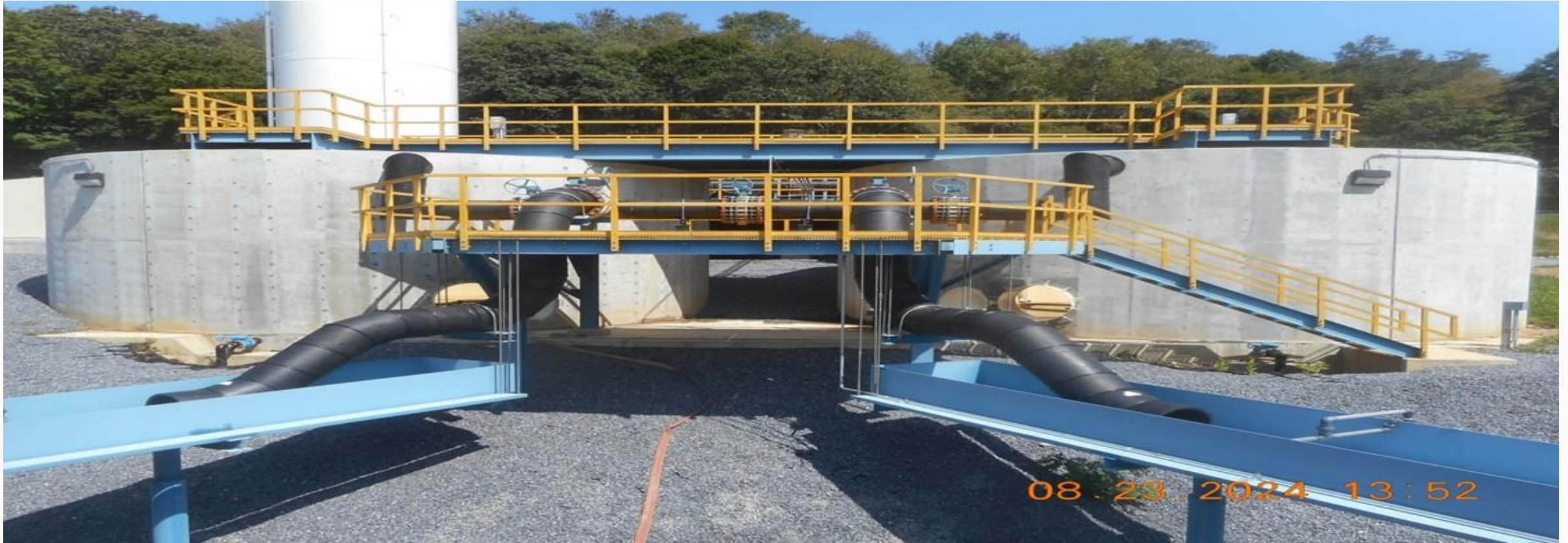
Reaction Tank Valve Platform and Flume to Clarifiers
