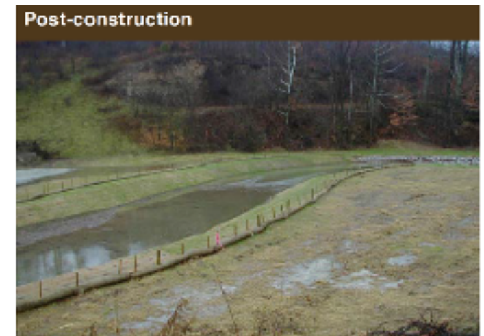
Completed natural channel stream Photo by Kaabe Shaw
