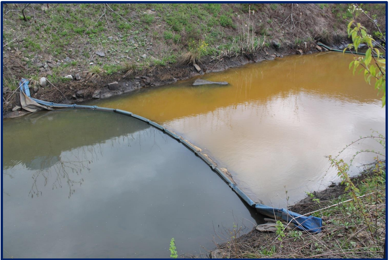
Example of windows not big enough to accommodate the flow and forcing water to flow under the baffle.
