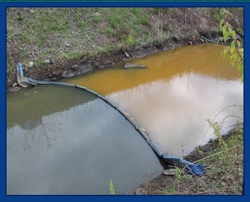
Example of windows not big enough to accommodate the flow and forcing water to flow under the baffle.
