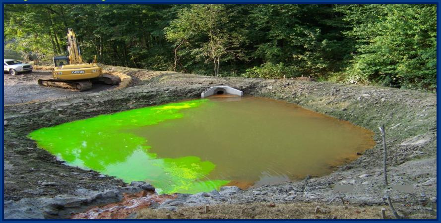
This next pond has a twist in regards to flow path influences. The water enters at the rear of the pond where I am taking the picture from. In addition, there is another source about a quarter of the way down the pond on the left side (black pipe) that is adding about 300 gpm's for a total flow of 550 gpm's. Does that flow sound familiar? If you guessed that this pond feeds into the first pond we looked at, you would be correct.
