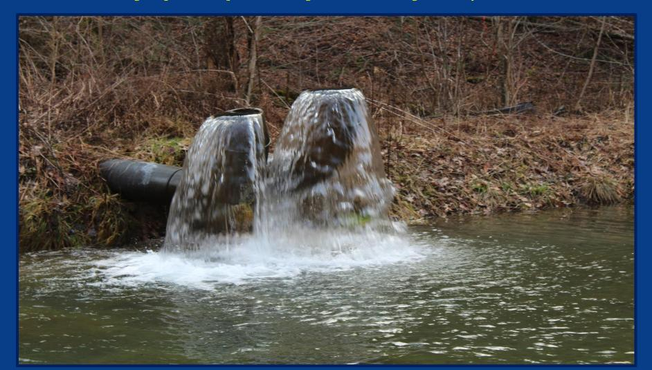
As this method might not always be possible, how about just piling a bunch of big rocks right at the entrance of the pond (energy dissipater) to break the flow path? Anyway, the manner in which the water enters your pond will help determine how successful you are in distributing the flow to obtain maximum retention time.
