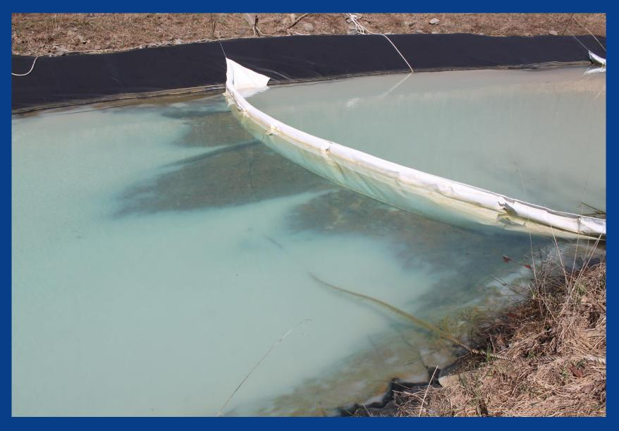
Since the windows in Surface Skim Baffles are about 6" below the surface, they also act to prevent oil or coal dust from exiting the pond.
