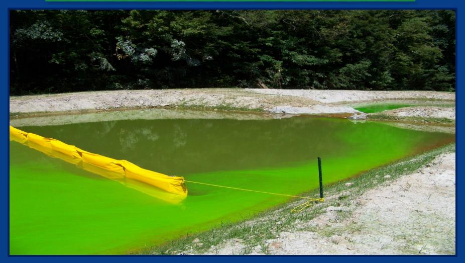
So, what do you think. Are ZigZag's the way to go? They lengthen the flow path but carry solids throughout the pond each time they sweep around the end of a curtain, and they fail to efficiently utilize the entire pond for sludge deposition and storage. If not ZigZag baffles then what?
