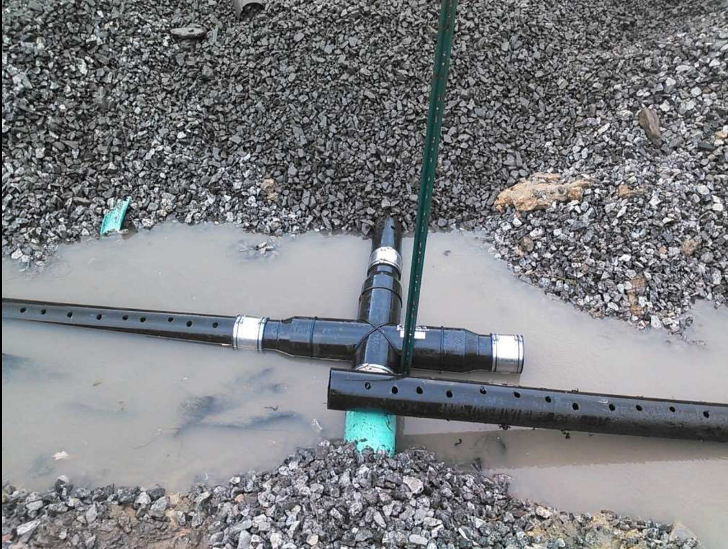
T-posts to mark pipe junctions
