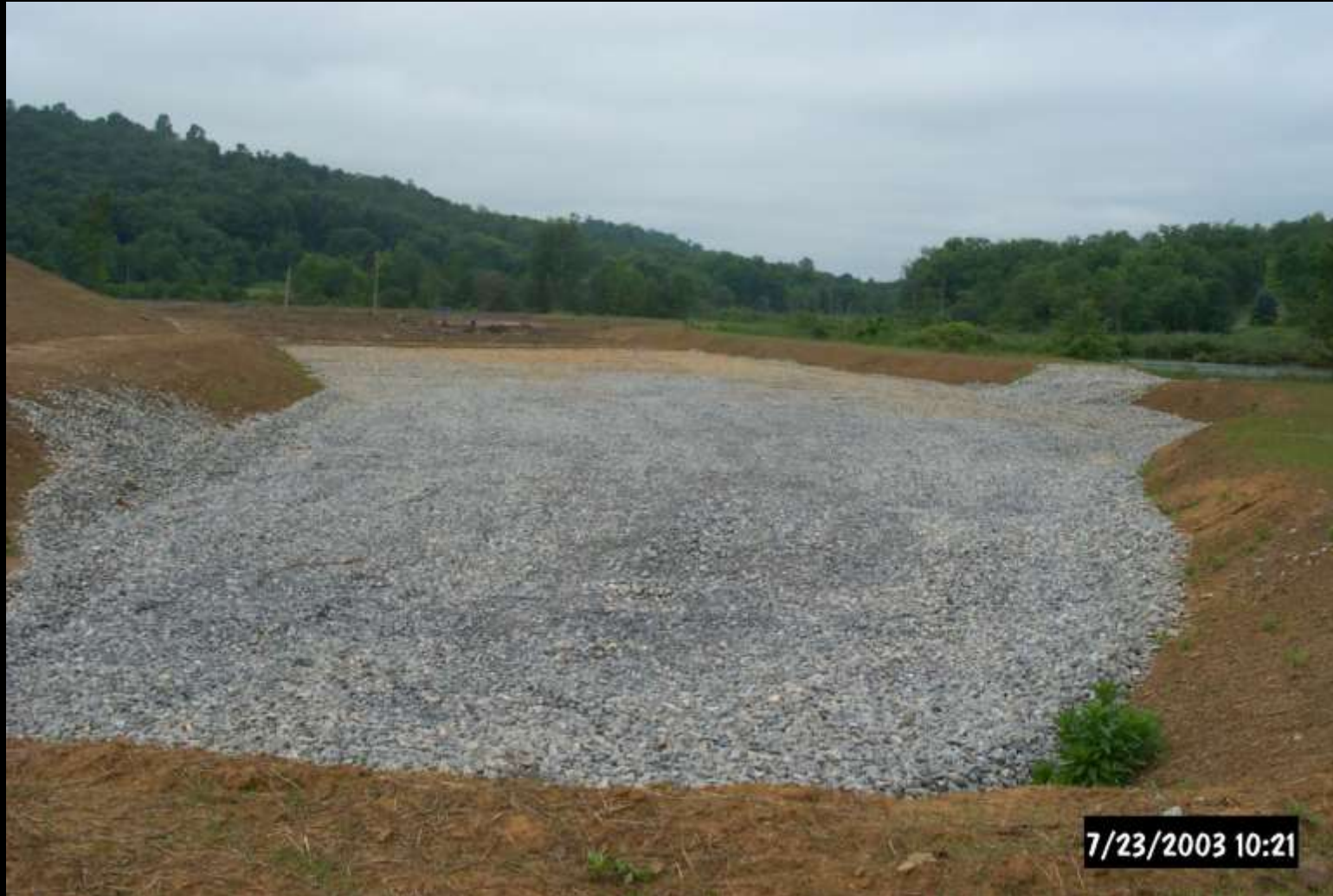
HFLB bed with perforated outlet header
