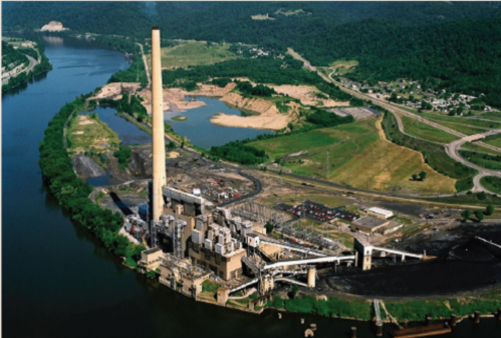
Future building site of the ethane cracker plant at the Big Run Gob Pile Project Site, Ohio
