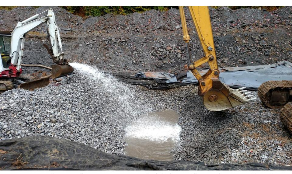
Limestone cleaning. The mini excavator on the left directed flow as the 315 on the right mixed the stone. Water flowed out of the bed through the flush pipes on the bottom.
