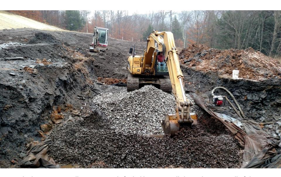
The limestone in Cell C was severely fouled but it was all cleaned. Moving all of the solids out of the bed was a challenge.
