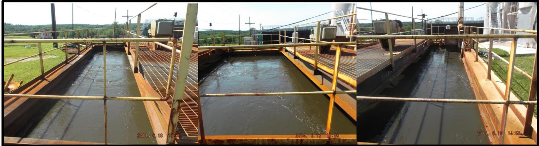
1. Dissolved Oxygen maintained  $> 2$  mg/L across Mixing Tank
