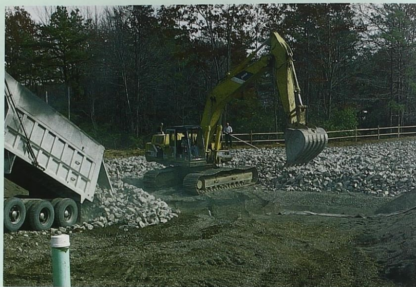
Figure 3. Construction of the limestone leach bed with limestone chips placed at the bottom overlain with large limestone rock. The 8-inch inlet pipe is the green pipe in the foreground.
