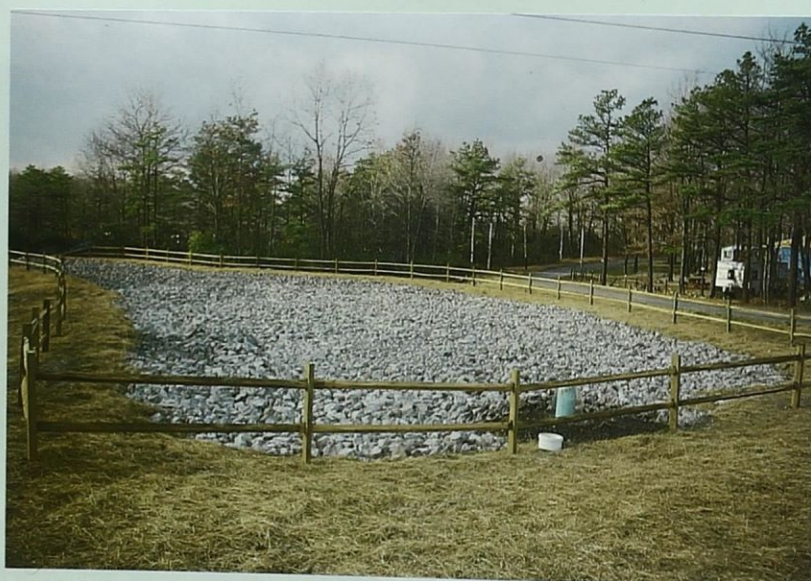
Figure 4. The leach bed inlet pipe in the foreground delivers approximately 100 to 120 gpm from the swimming lake into the leach bed. The leach bed is about 50 feet wide, 4 feet deep, and 200 feet long. The split rail fence restricts access to the leach bed.
