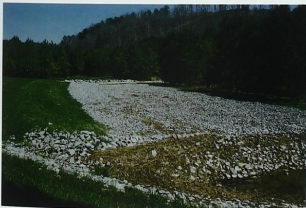
Figure 1. A limestone leach bed constructed under the Clean Streams Initiative in the Cane Creek watershed of Alabama.
