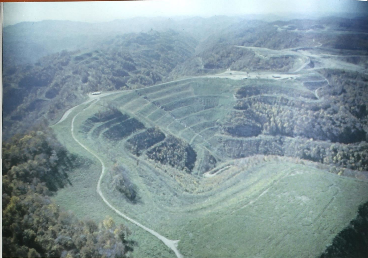
The fill is constructed to generally follow the contours of the hollow, as evidenced by this aerial view of a Buffalo Mining Co. operation in Logan County.
