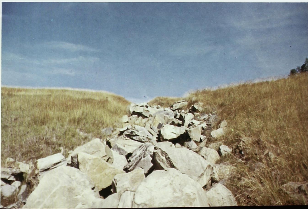
The chimney drain rock core, which extends from the surface to the valley floor, is the key to West Virginia style valley fill construction.
