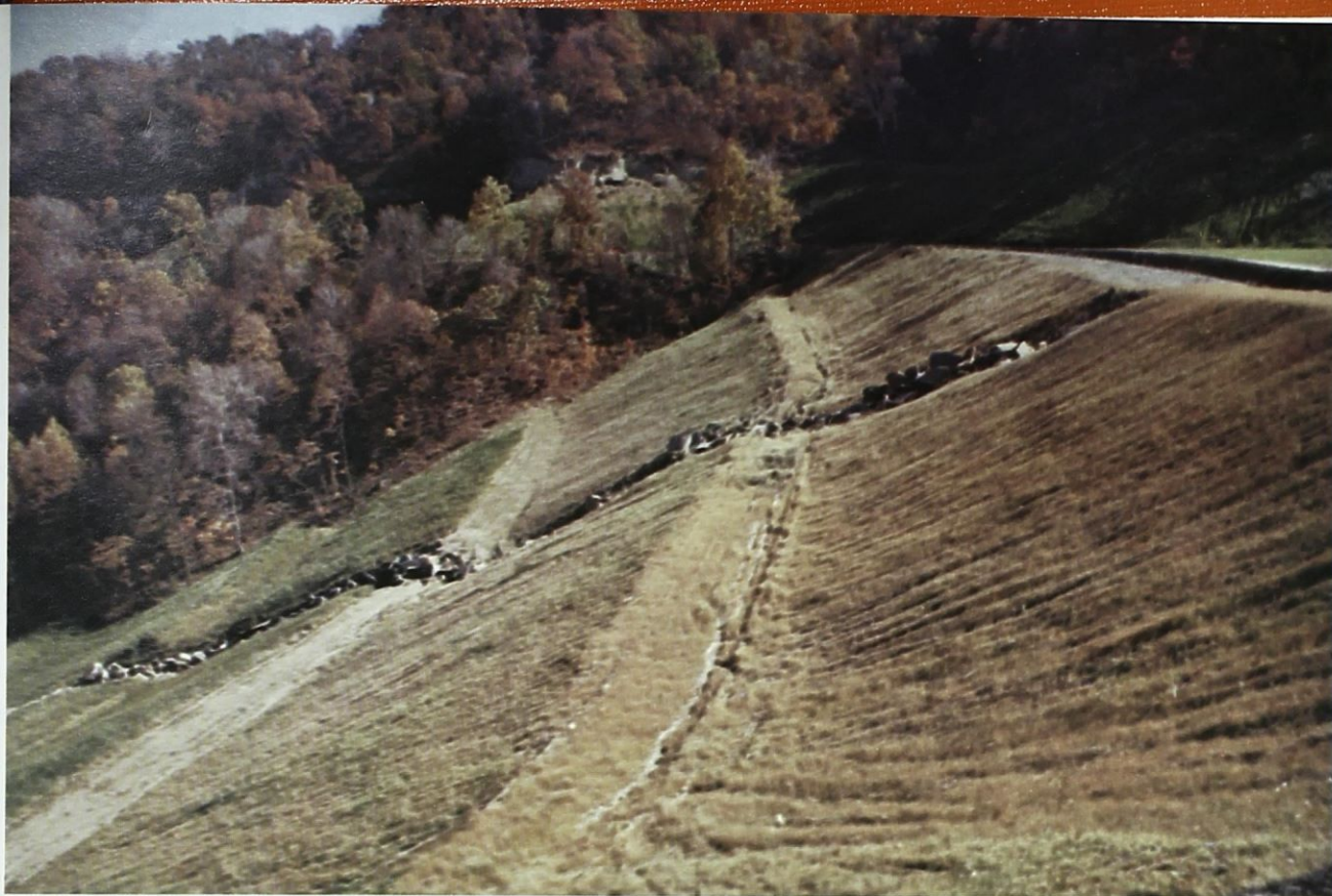
The terraced effect of the completed fill diverts surface water to the rock core.
