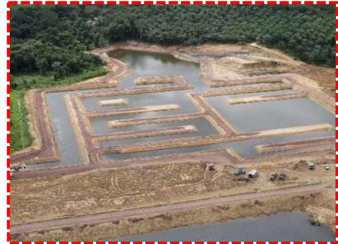
The mine water discharge processed in the settling pond is exceeding large → high consumption of chemical coagulant
