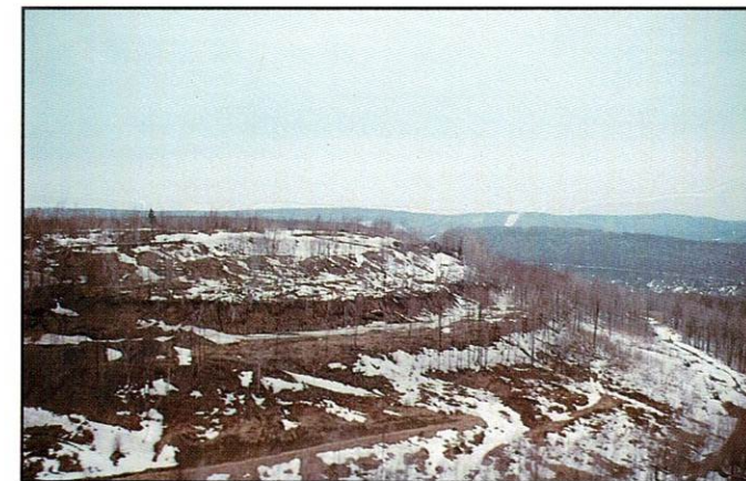
The Fairfax site was a 100 acre remining site in West Virginia. The previous mining operation left highwalls, coal refuse on the surface and extensive underground workings. Moderately acid water was found on the site. (Note the power line right-of-way in the background). Picture taken March, 1985.
