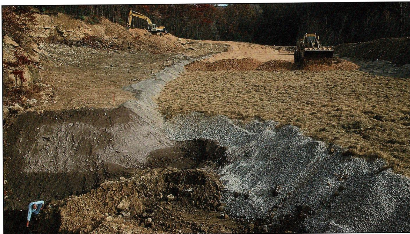
The anoxic limestone drain was engineered from water properties data gathered over a six month period.
