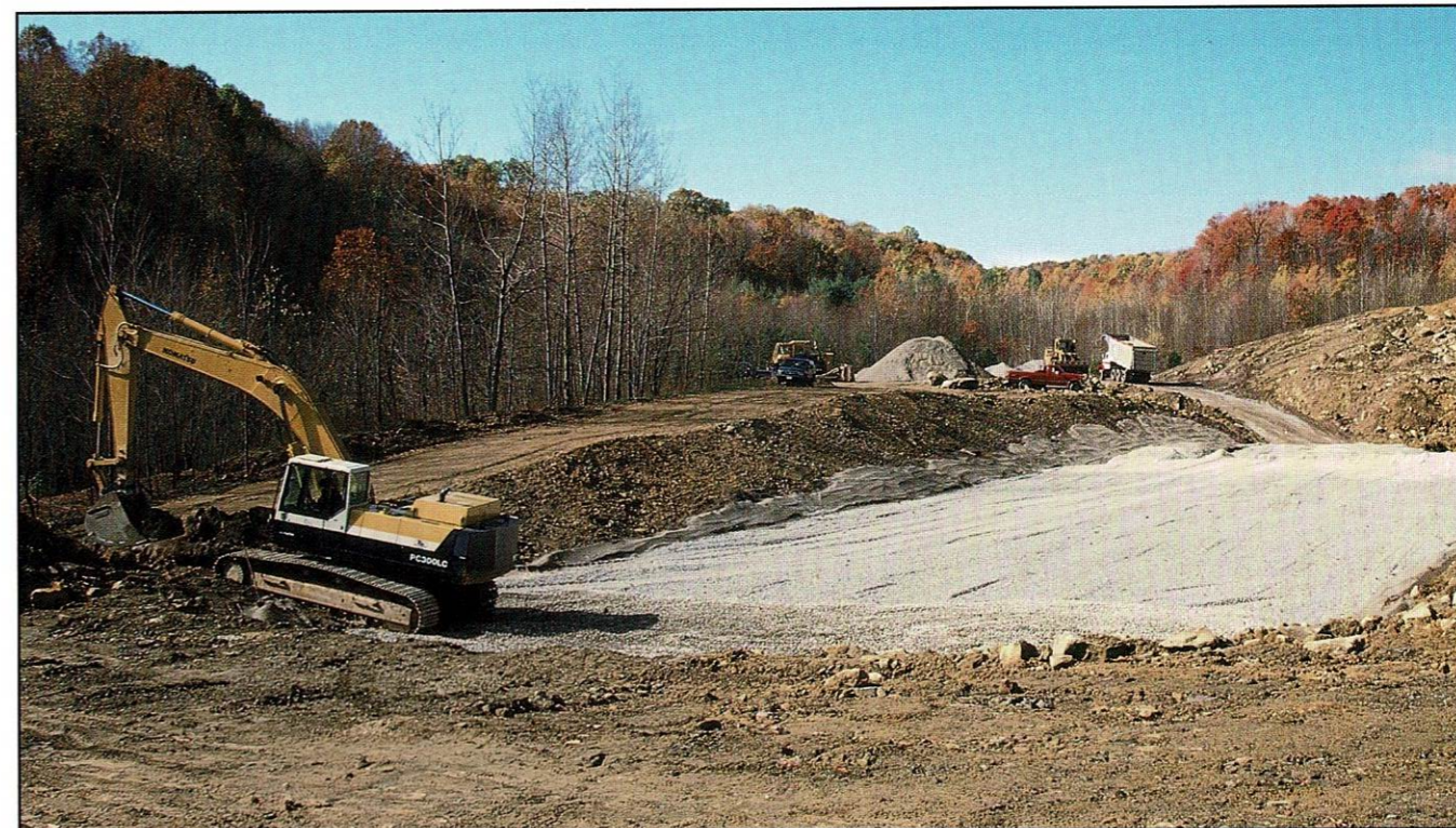
Phase 1 at Greens Run involved construction of an anoxic limestone drain to neutralize an acid seep from an old highwall.
