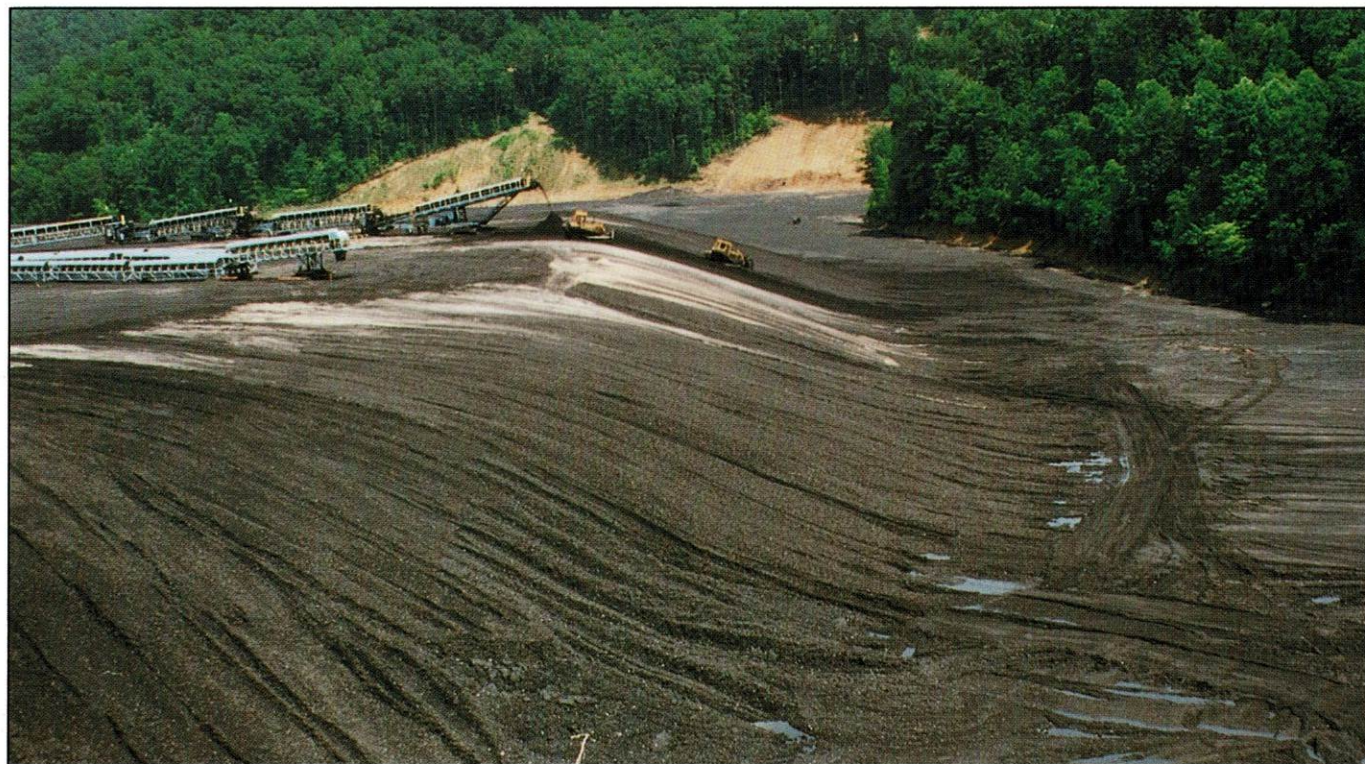
At Brooks Run Coal Co., a limestone additive is mixed with refuse continually as the fill is constructed.
