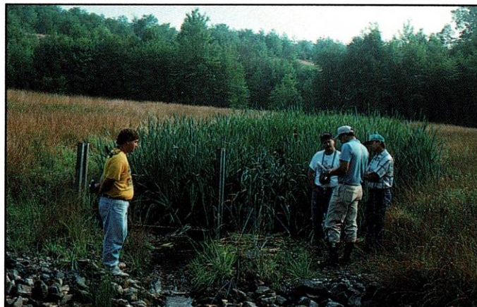
Constructed wetlands are especially practical when dealing with acid mine drainage from abandoned mine lands. The wetland provides some treatment with little or no maintenance costs.
