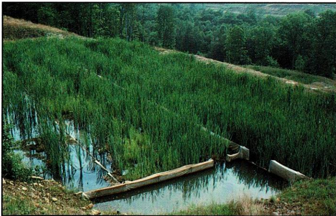
Residence time in wetlands is important to maximize water contact with the wetland substrate where microbial transformations and oxidation/reduction reactions occur. Sometimes baffles are necessary to facilitate water movement through the wetland.
