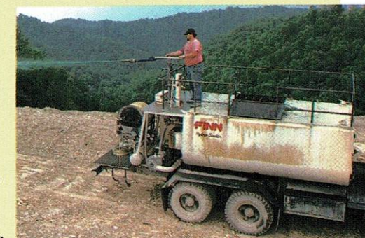
A mix of fertilizer, seed and mulch is sprayed on the site.
