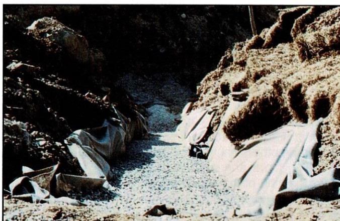
Anoxic limestone drains are buried cells of limestone. When properly constructed and with the right type of water, alkalinity can be introduced into the water and help passively treat acid mine drainage.
