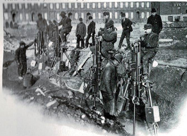
Rand Rock Drills at work on the Site of the Pennsylvania Railroad Terminal, Thirty-fourth Street and Seventh Avenue, New York
