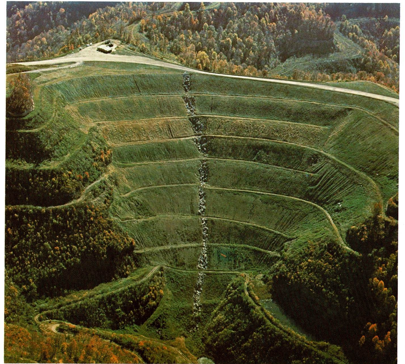
Buffalo Mining Co. demonstrates that valley fills can be of quite an imposing size which has proved especially beneficial to mountaintop operations.
