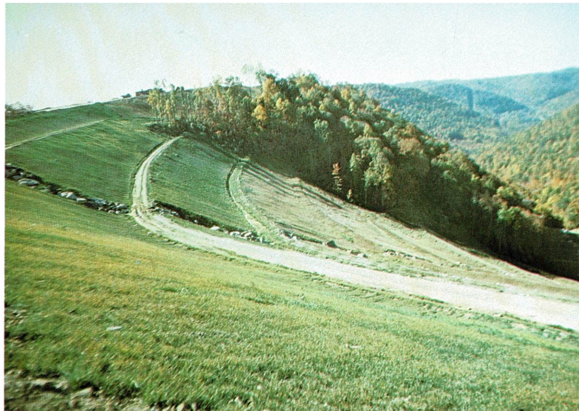
Terraces are slanted toward the rock core which prevents any significant flow of water across the face of the fill.
