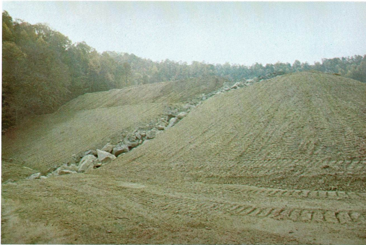
Quick and complete revegetation not only enhances the appearance of a reclaimed site, but prevents a myriad of problems which could otherwise arise from the unchecked flow of water over bare earth. Effective revegetation is even more critical in areas like steep sloped Logan County, where these shots were taken at the same site, just over six weeks apart.
