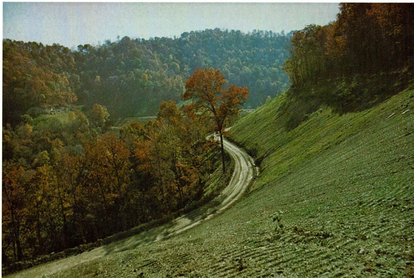
Even in its unvegetated state, the advantage of the controlled placement of overburden materials that haulback offers are apparent.
