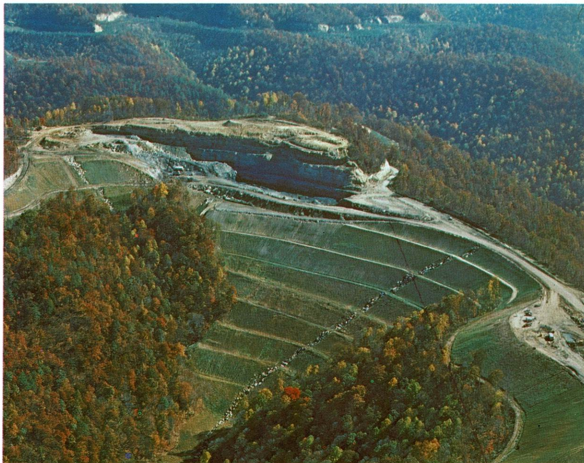
The stability and effectiveness of a properly constructed fill is such that mining can be carried out on adjacent acreage, as on this Cedar Coal site.
