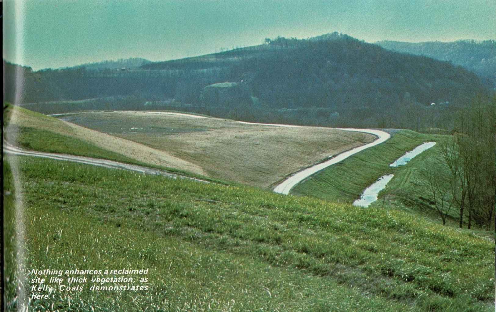
King Knob presented a good example of West Virginia's innovative approach to valleyfill construction. The rock core shown here extends to the valley floor.
