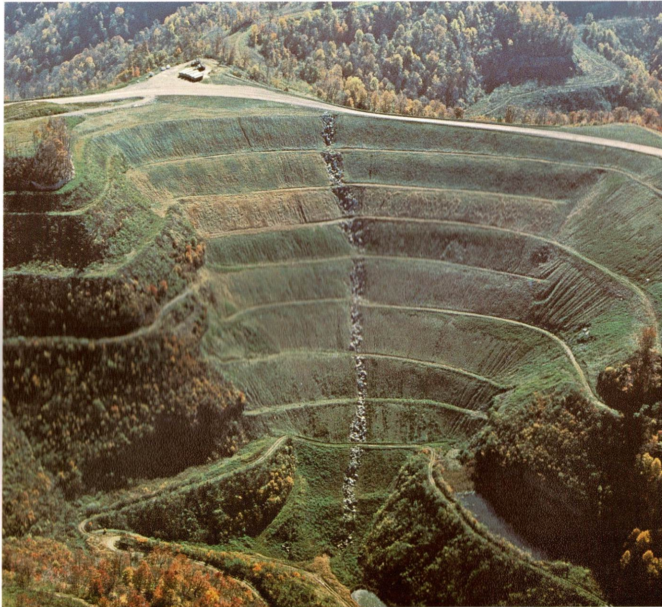
This photo, and the comments which accompanied it, created quite a stir following publication of our Spring issue. Shown is a rock-core chimney drain fill constructed by Buffalo Mining Co. in Logan County.
