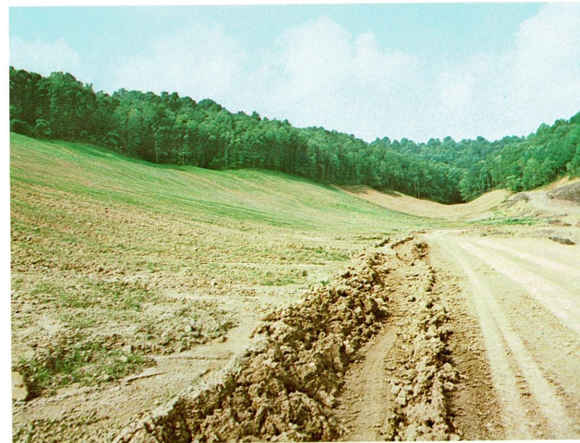
The Galloway Co., Inc., also working in Upshur County, is returning this land to its original contour with an intended post mining use as pasture.
