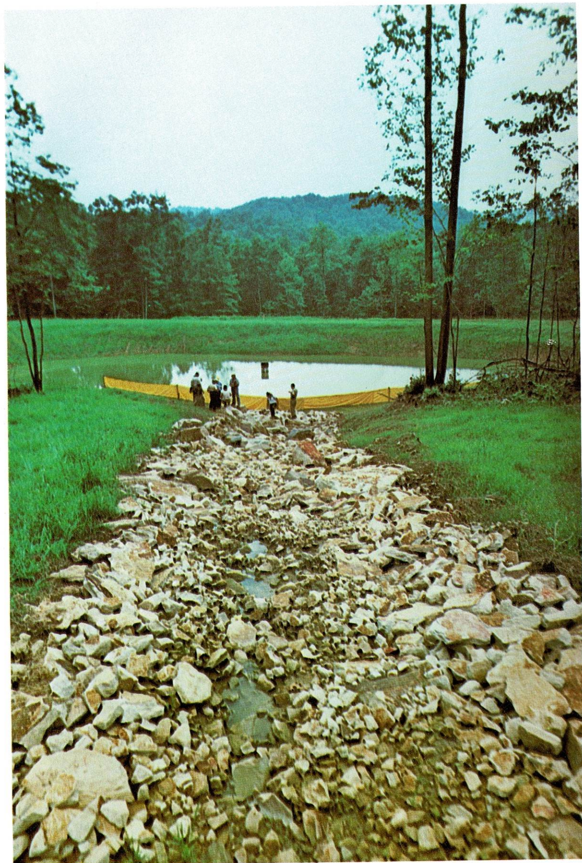
La Rosa Fuel Co., Inc. uses rip-rap drainage (foreground) and a canvass "baffle" to aid in sediment control.
