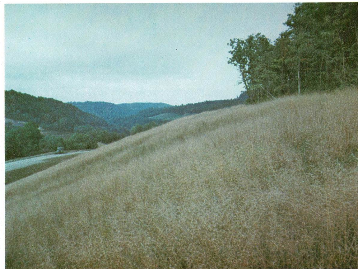
This Sterling Smokeless job, also in Raleigh County, utilizes the haulback techniques to achieve concurrent reclamation. Coal extraction is ongoing just a few hundred yards away.
