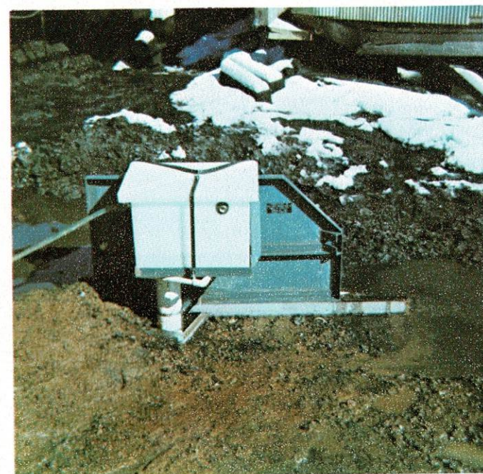
Soda ash briquettes are used to neutralize acid water through units such as the one pictured here.
