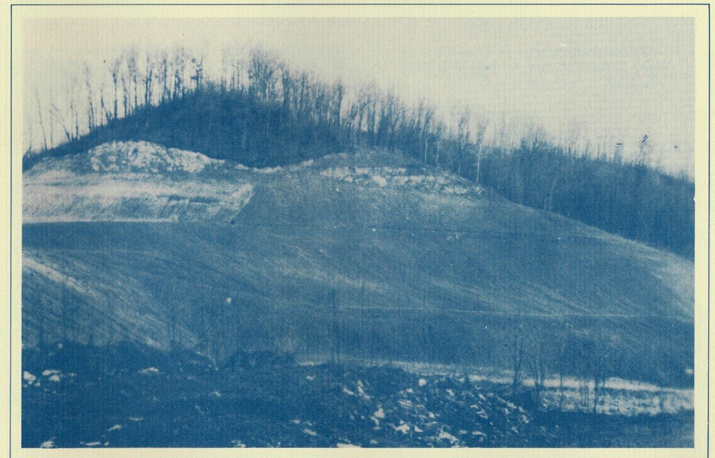
Figure 3—Overburden Replacement At A Former Mine Site Near Welch, West Virginia
