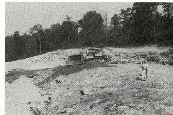
Valley Camp is top soiling all of its surface mine operations. On this job near Witcher Creek a bulldozer is working to put the good material back on the top. This method of regrading has greatly improved the revegetation program and helped the company win a reclamation award from the West Virginia Surface Mining and Reclamation Association.
