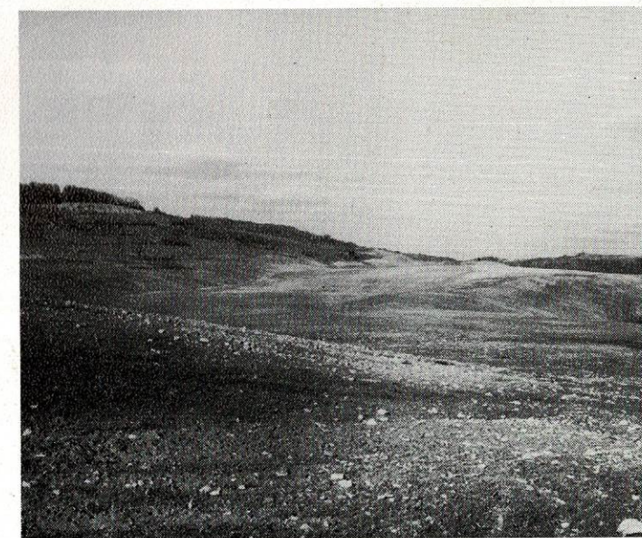
In many instances the original top soil may not be the best material for revegetation. In this case a selected sub-soil will be segregated and replaced back to the surface.
