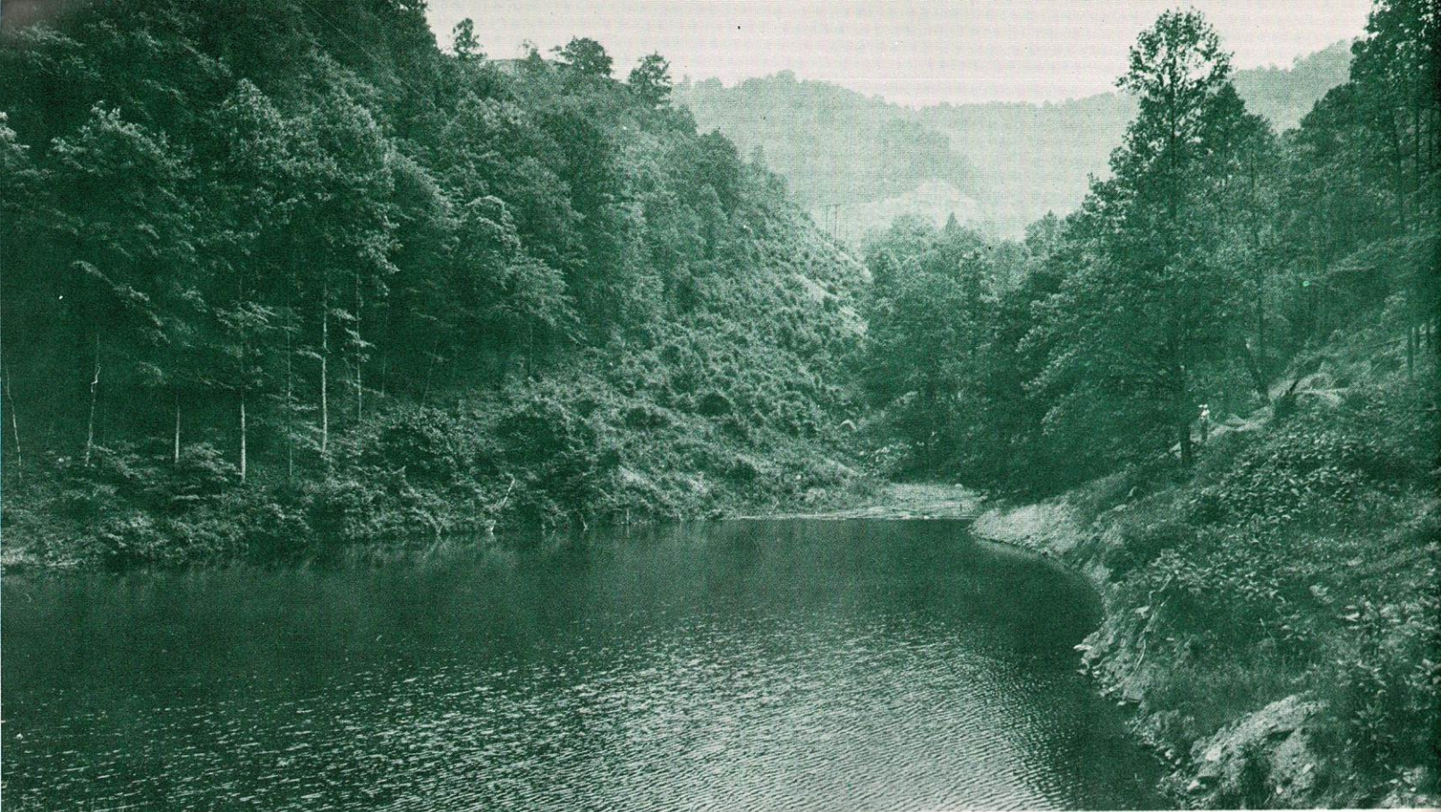
In accordance with the provisions of the 1971 Surface Mining Act complete drainage systems and sedimentation ponds must be included in the mining plan. Water flowing into the pond above circulates allowing the silt particles time to settle to the bottom before the water runs out into the stream.
