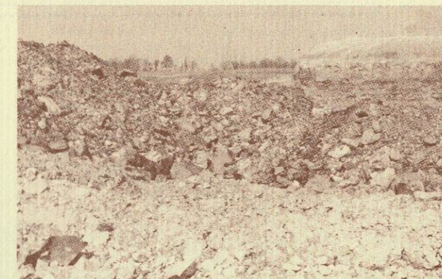
Figure 9: Stacked spoil prior to recontouring; light material in foreground is acid-free and dark material in background contains acid.
