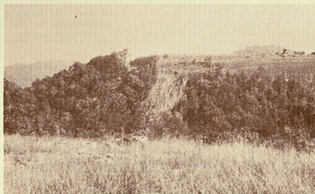
Figure 2: An outslope that has had a slide.
