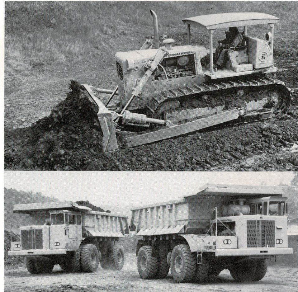
LEVELING UP TOP SOIL OVER SURFACE MINE IS INTERNATIONAL'S TD-25C. PH-180 PAYHAULERS HAUL TOP SOIL FROM BORROW PIT. BOTH ARE PRODUCTION COAL MACHINES DOUBLING AS PRODUCTION RECLAMATION MACHINES.
