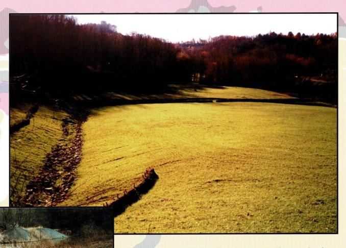
This four-acre project, about two miles north of Clarksburg, addressed problems including eroding coal refuse, open and collapsed deep mine portals, mine subsidence impounded water and acid mine drainage. A total of 7,700 cubic yards of coal refuse was excavated and regraded, covered with soil and revegetated the entire site. The project was completed in the fall of 2001.
