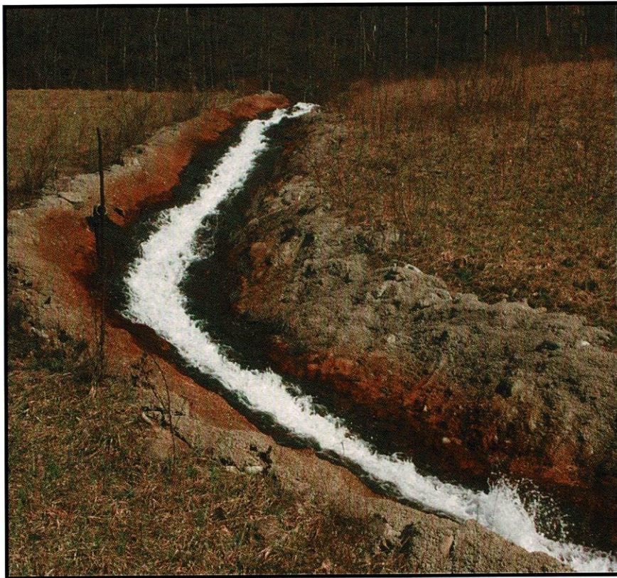
Site 15 is a reclaimed site, done by the WV AML program. This riprapped grouted channel conveys discharge down the hill to Muddy Creek.
