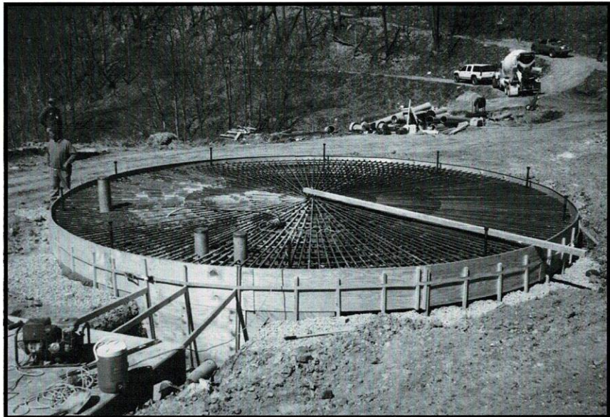
A foundation for a water tank is being constructed on Buffalo Mountain as a part of the Pigeon Creek project in Mingo County. This particular tank cost about $210,000 and will hold 263,000 gallons. Water tanks provide head pressure for the system.
