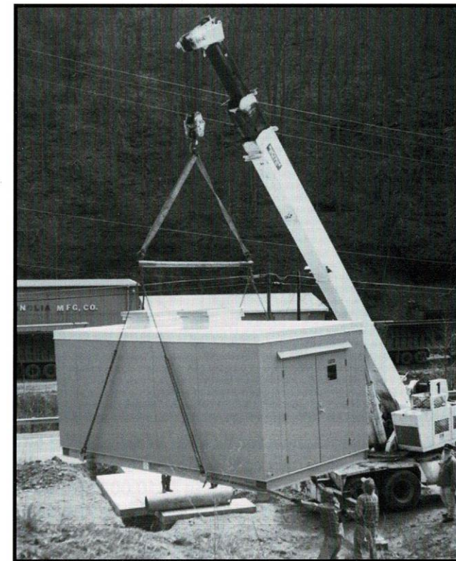
Workers ease a pump station in place during construction in Mingo County. Pump stations such as this one provide pressure to fill up water tanks. Cost of this station was $195,000.
