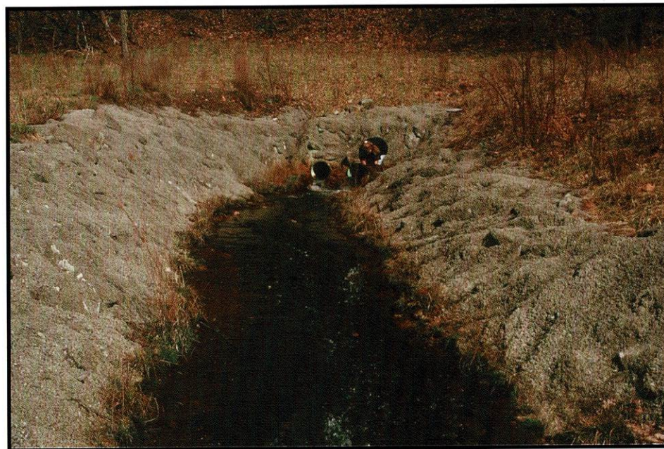
The pipes at Site 15 extend back into the mine through the seal placed at the portal, thereby allowing flow out of the mine.
