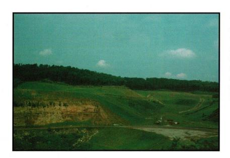
This valley fill is one of the early fills where "green" sandstone was placed on the surface for riprap. As a result of incorrect knowledge of the material's acid-producing potential, a small amount of chemical treatment is needed before this water can be discharged.
