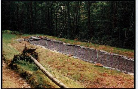
To achieve optimum metal removal, the size of the bed should be such size to give the AMD a 3-day retention time.
