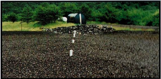
Once the treatment bed is constructed, limestone added and filled with water, then both solid inoculum (bacteria coating limestone grown in the laboratory) and liquid inoculum of bacteria are added.
