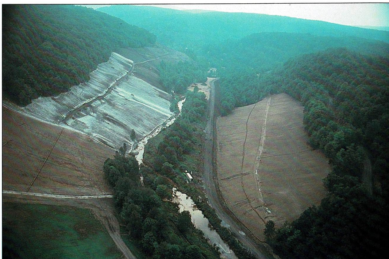
Picture 6. Aerial photograph from nearly the same point as picture 5. The highwalls were eliminated on the left and the refuse pile has been regraded on the right. The ALD/Wetland system is located on the right side of the road and continues around the corner at the top of the picture. This picture was taken in September 1993.
