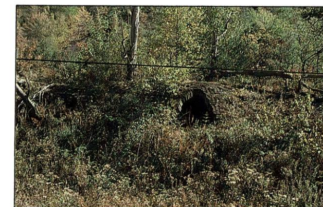
Picture 1. One of the 600 potential 2-ton coke ovens on the Douglas Highwall AML Project. Reclamation of the site left most of the ovens intact.
