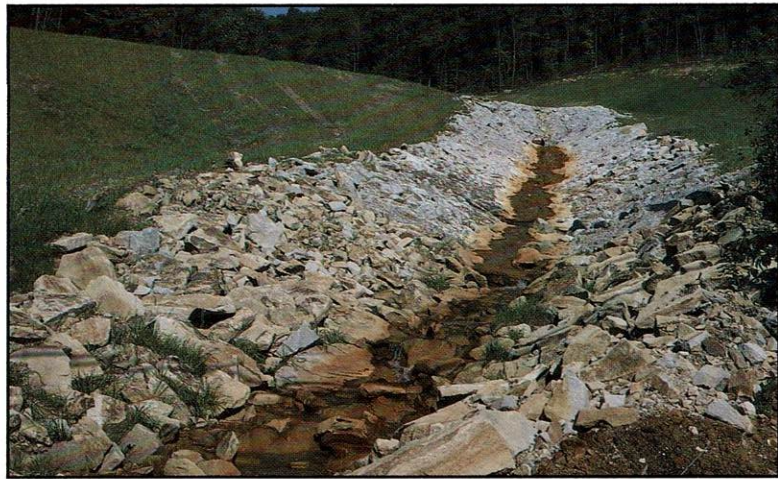
Figure 1. Many open limestone channels which convey acid mine drainage are armored by iron precipitates. Many people assume that armored limestone will provide no treatment to the acid drainage.
