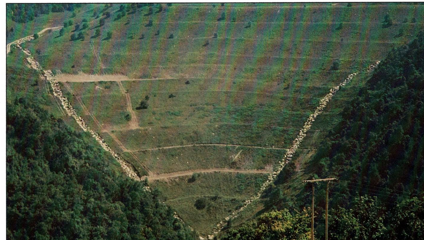
Like its sister mine, Ruffner, Wylo uses end dump valley fills for excess overburden disposal.
