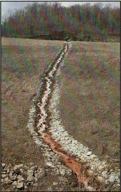
Figure 2. The open limestone channel on the Brownton AML site. This channel is about 500 ft long and is covered with ferric hydroxides.
