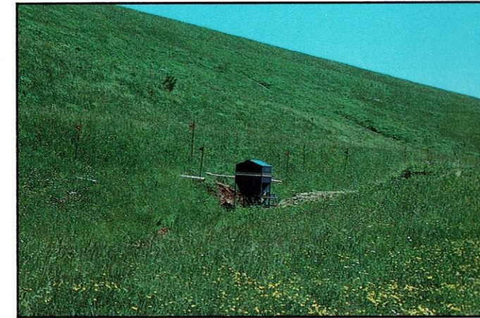
Water from a pipe is then introduced into the unit to power the water wheel, which then turns a screw feeder in the hopper. Approximately 2000 pounds of pelleted quicklime can be loaded into the hopper.
