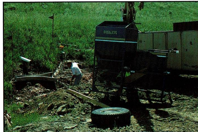
Some site preparation is normally required to make/build a level place for the Aquafix Machine to set. It usually straddles the stream.
