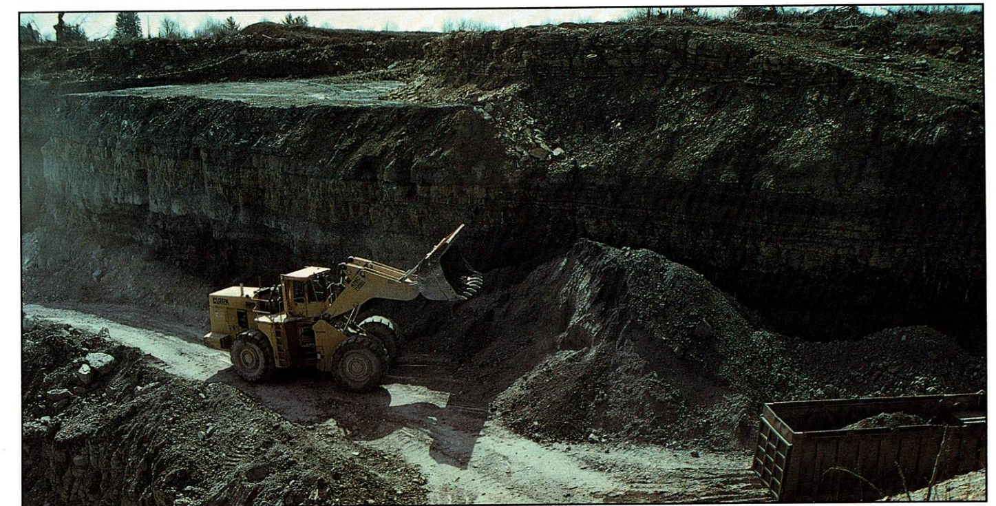
Figure 2. Alkaline red shale from the Bakerstown coal surface mine was loaded into coal trucks and hauled to the Upper Freeport job.
