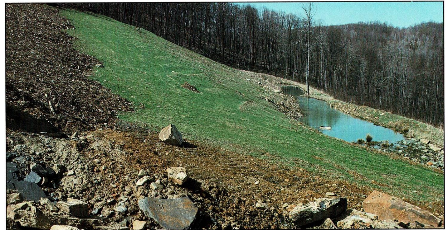
Figure 4. With the addition of alkaline material on the pavement and to the soil surface after grading, water quality on the site has been greatly enhanced. The surface reining operation daylighted old deep mines and eliminated AMD discharging from the portals.
