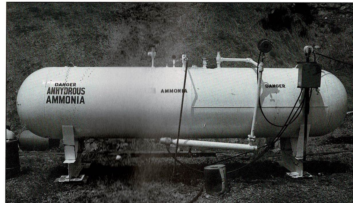
Figure 5 - An ammonia tank equipped with a vaporizer. The vaporizer is a heating element which helps maintain a consistent pressure in the tank for uniform vapor dispensing.
