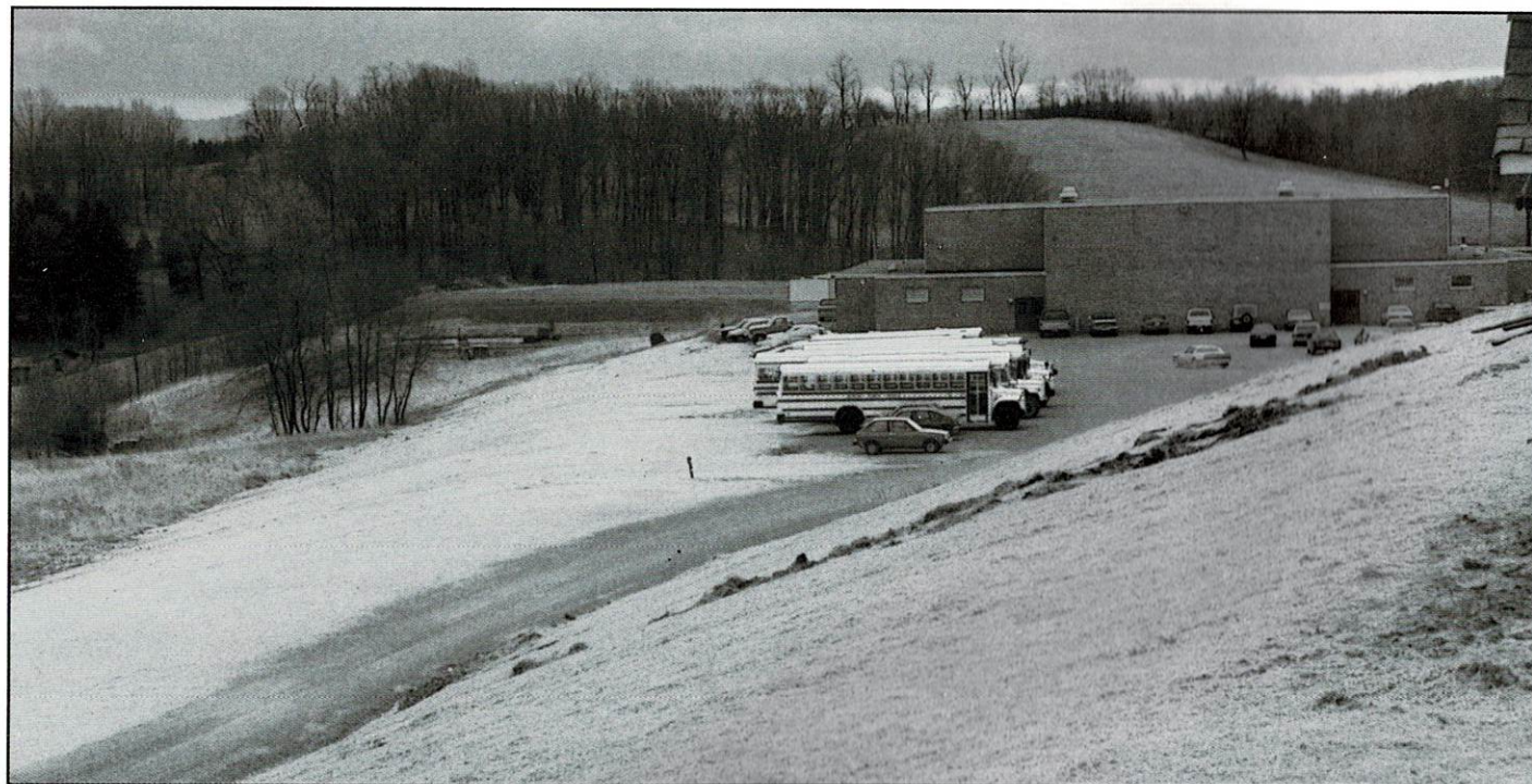
Fill dirt from the construction site provided material for a contoured bank behind the school.
