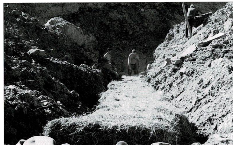
Figure 2. Hay bales were placed on top of the filter fabric lined trench filled with limestone.
