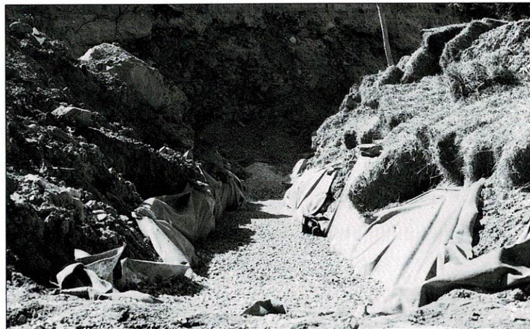
Figure 1. Excavation of the trench was followed by placing filter fabric in the trench, and then filling the trench with limestone.
