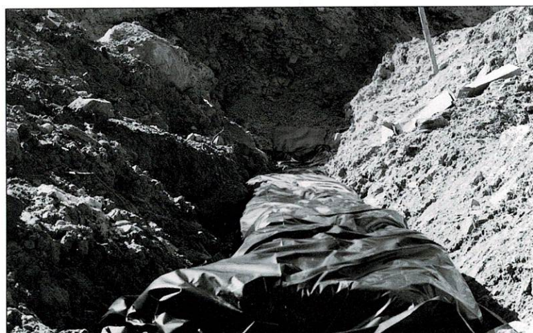
Figure 3. The limestone and hay in the trench were covered with plastic.
