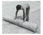
Starting at the top of the slope to be covered just unroll the Blanket. The Blanket should never be stretched so that contact with the soil can be maintained. Follow the simple instructions included with each roll
