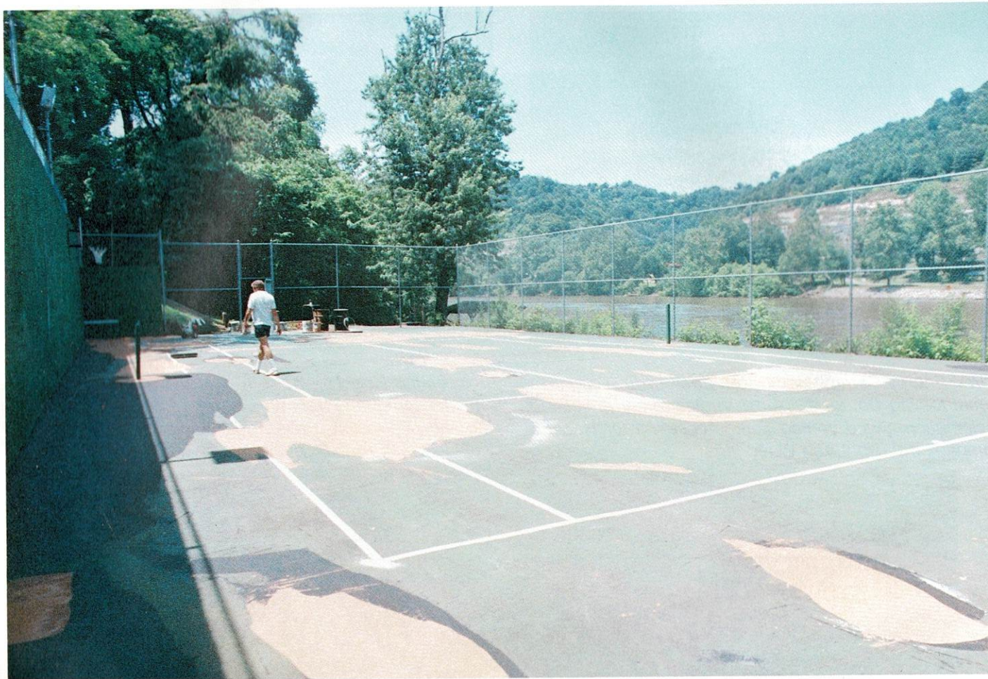
Bob Martin checks the progress of patchwork prior to resurfacing.
