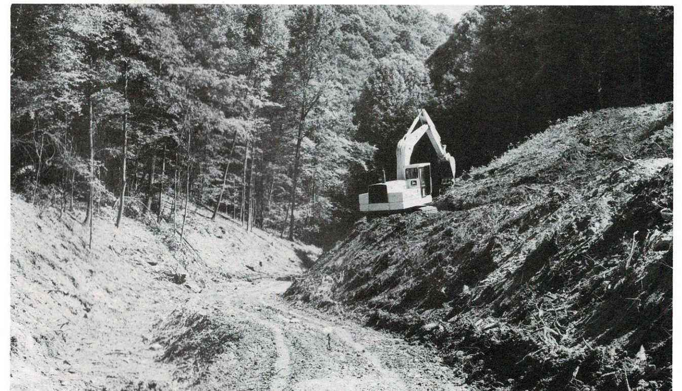
Backhoe excavating for a drainage control pond in Sugarcamp Hollow.
