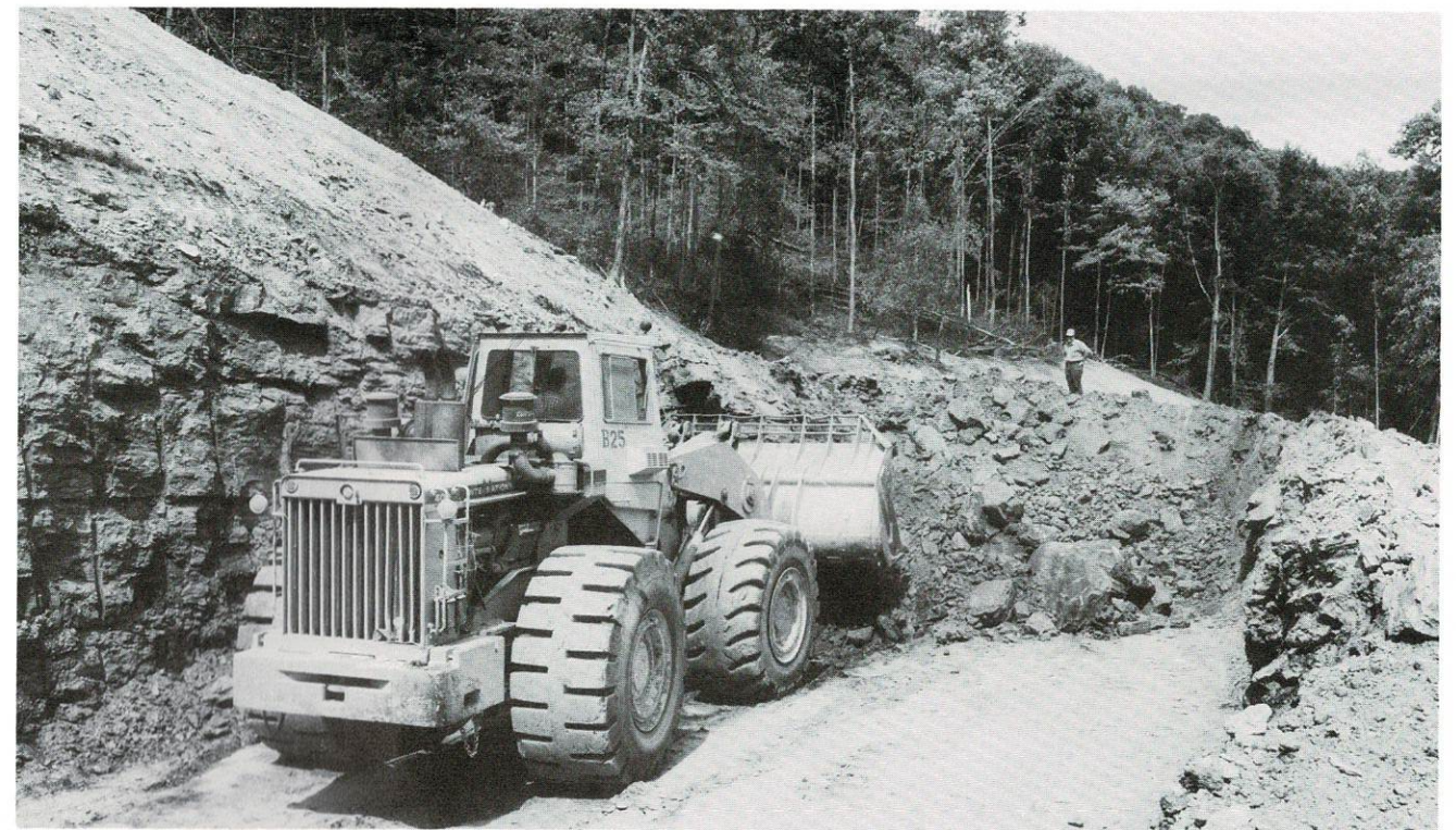
Front-end loader clearing the main access roadway.
