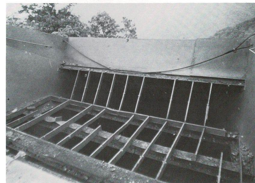
Armco demonstrated its unique coal chute to tour participants. The 33 inch diameter pipe conveys coal from the surface mine on top of the mountain down to the deep mine site, an almost vertical distance of 1700 feet. The chute has proved to be advantageous in terms of speed, safety and economy.
