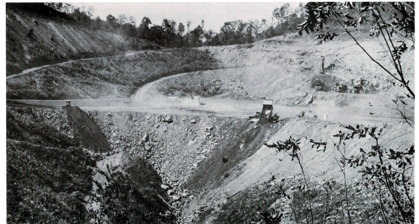
Initiation of dumping. Note the selective placement with finer material placed at the sides and coarser material in the center.
