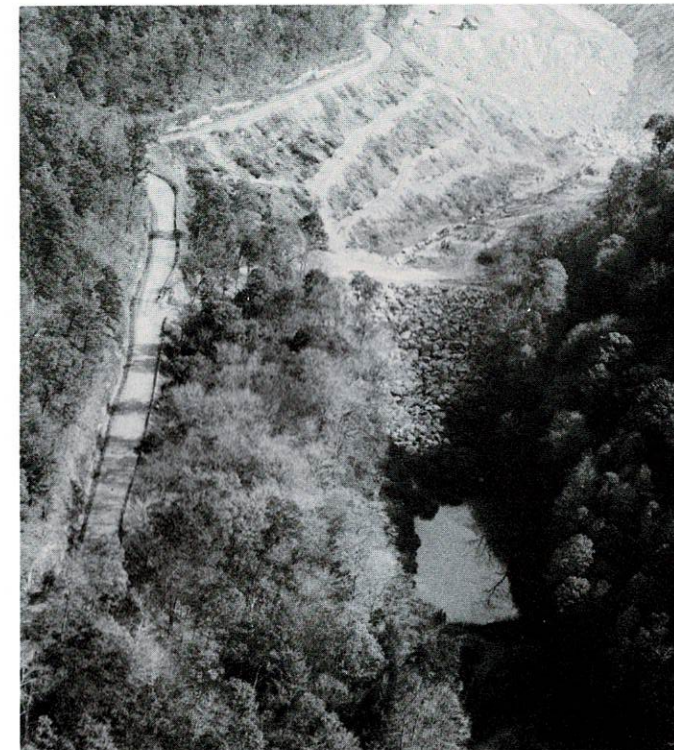
Toe dam for sediment control and stability of fill. Note the conventional sediment pond below the toe dam.
