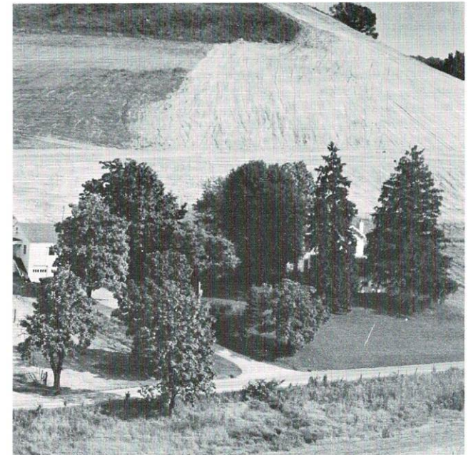
A closer look shows just how steep the hillside is even after mining. The highwall was eliminated here by blasting it down from the top, then grading. The last few acres at the right were just being prepared for seeding when this photo was taken in August.
