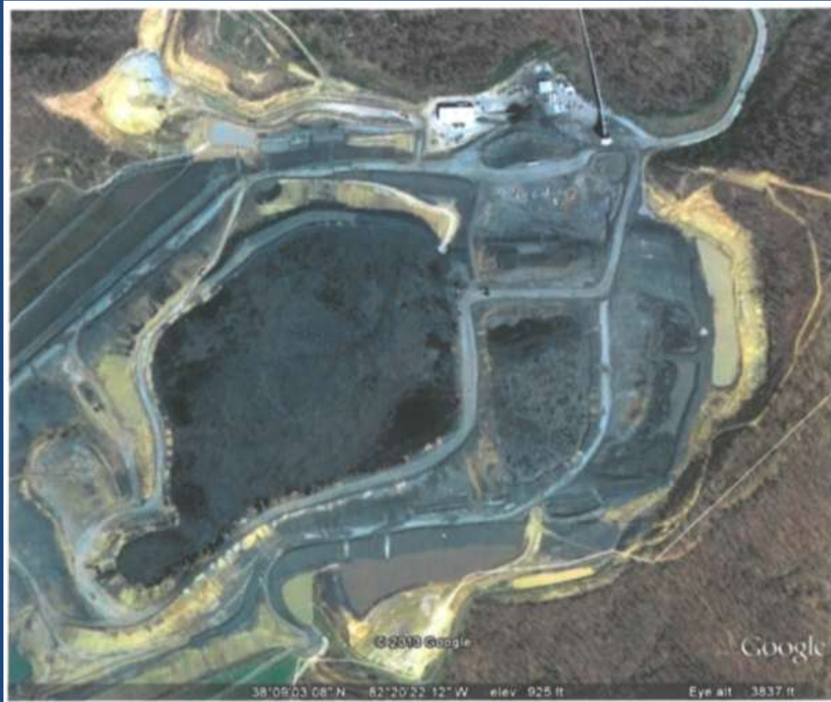
Overview of the Trace Branch Impoundment. 30 acre pool, center left. 5 acre pool, lower right from 30 acre pool.
