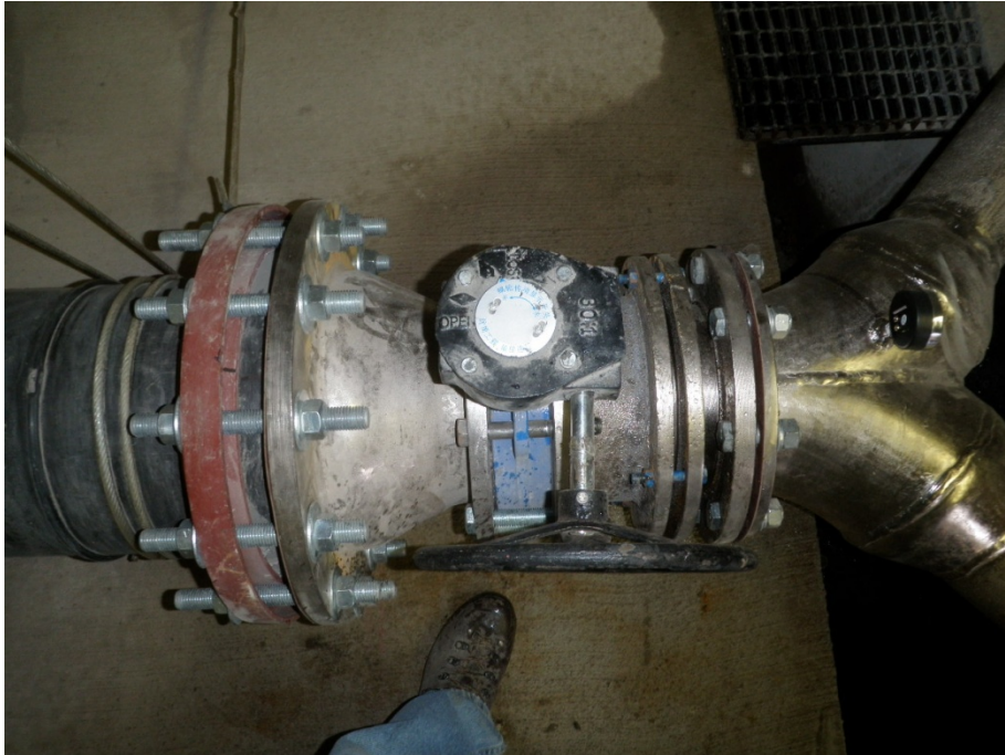
Figure 4. A portion of the powerhouse penstock components
