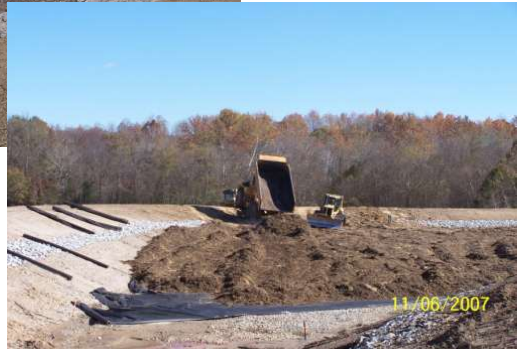
Under Drain Construction
