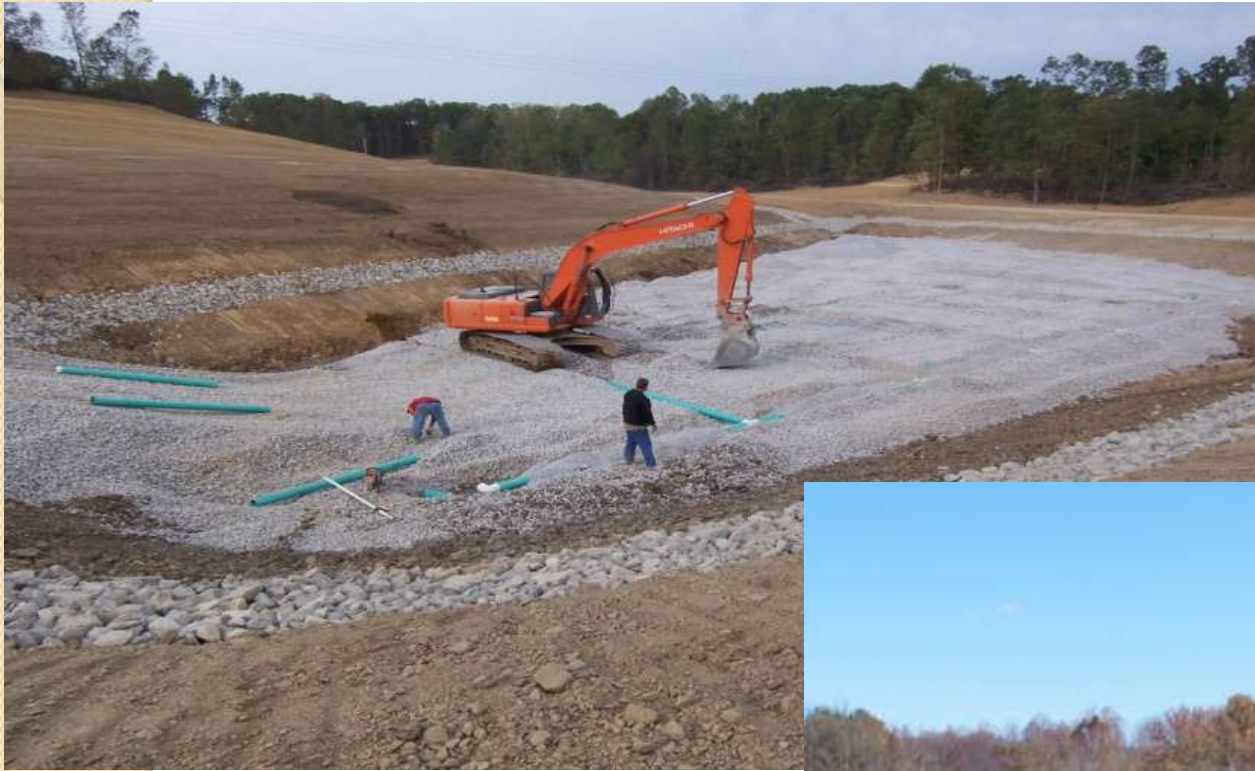
Under Drain Construction
